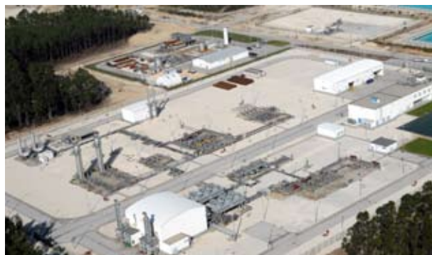
General View of the Gas Station
