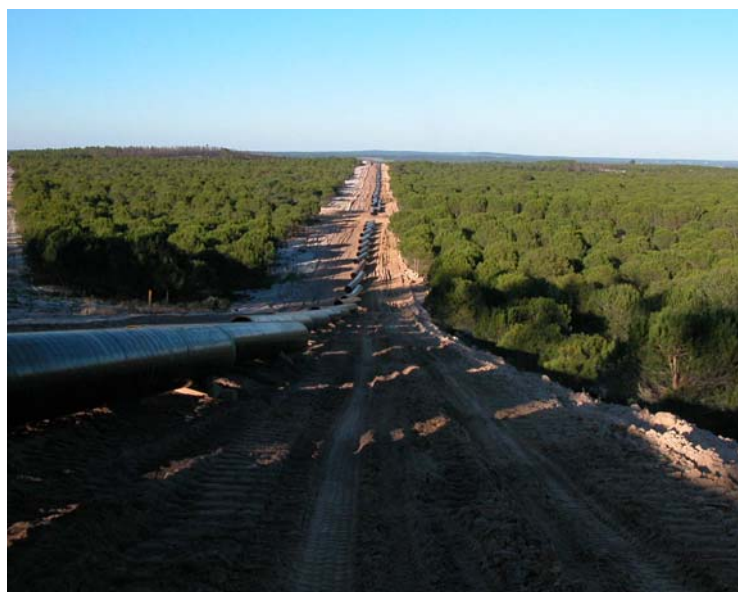
Construction of pipeline
