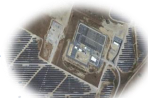
150/60 kV Ourique substation
