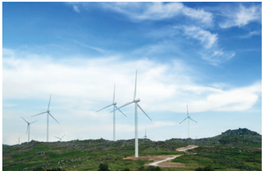
Wind farm of S. Macário II: as of June 3rd, 2011 it ceased to have limitations on its power connection, following a restructuring of the network topology, allowing to redirect its output towards the 60 kV of the Carrapatelo substation instead of the 60 kV of the Torrão substation.
