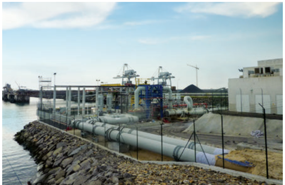
New sea water intake – Sines.
