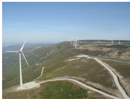
Malhanito Wind farm (60 kV connection at the REN Tavira Substation)
