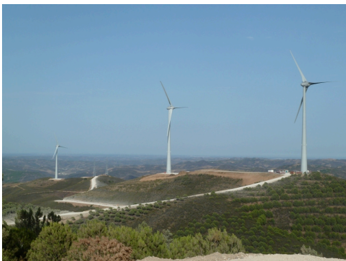
Malhanito Wind farm (60 kV connection at the REN Tavira Substation)
